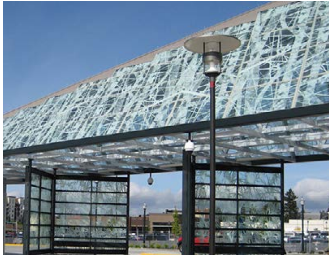
Fritted glass pattern panels Artist: Julie Berger Burien Transit Shelter, Burien, WA
